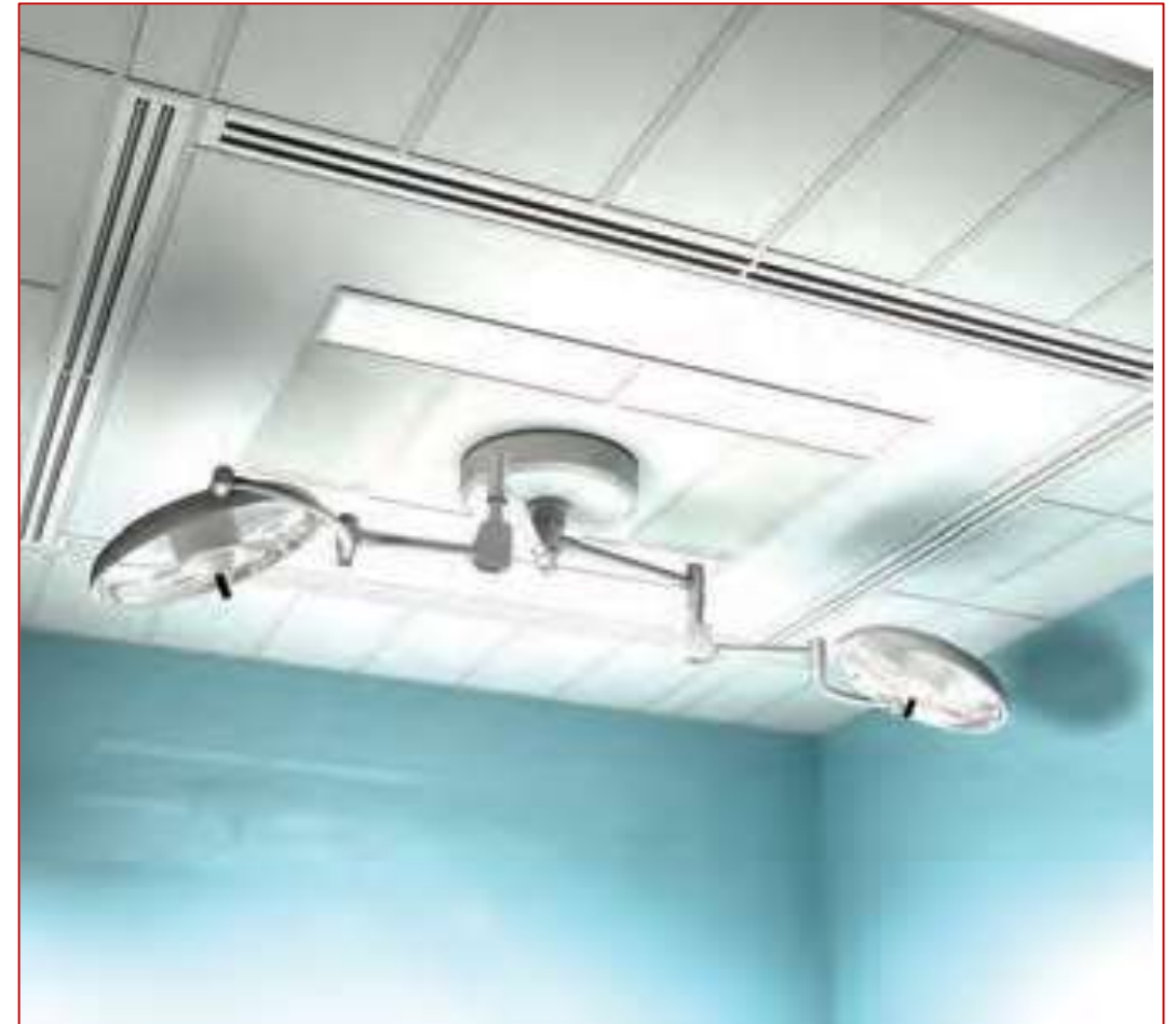
Air Curtain System 18
